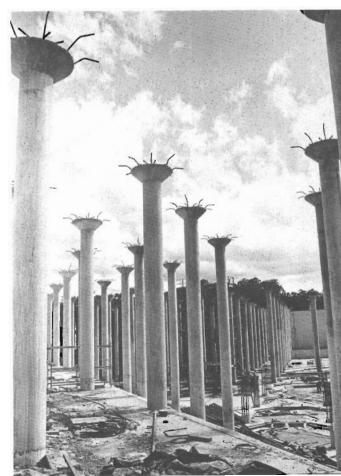
Support columns for the roof of the Sugarloaf Reservoir clear the water storage which will have a capacity of 200 megalitres. Melbourne and Metropolitan Board of Works
